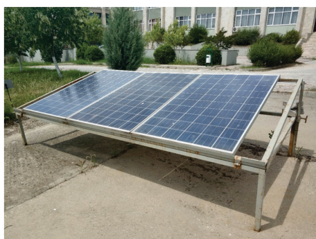
Fig. 1. Solar energy system installation
